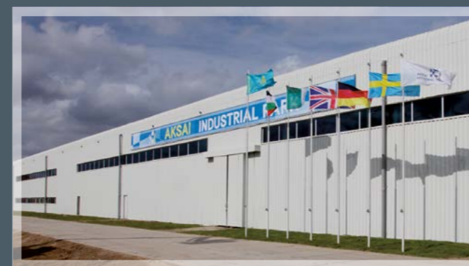
Sferova was selected to take part in the Aksai Industrial Park (AIP) Sferova Kazakhstan can manage assembling, testing, painting and after sales activities.
