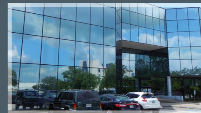
Sferova set up a representative and commercial office in Houston (Texas) in order to start close relationships with major US EPC's and End Users.
